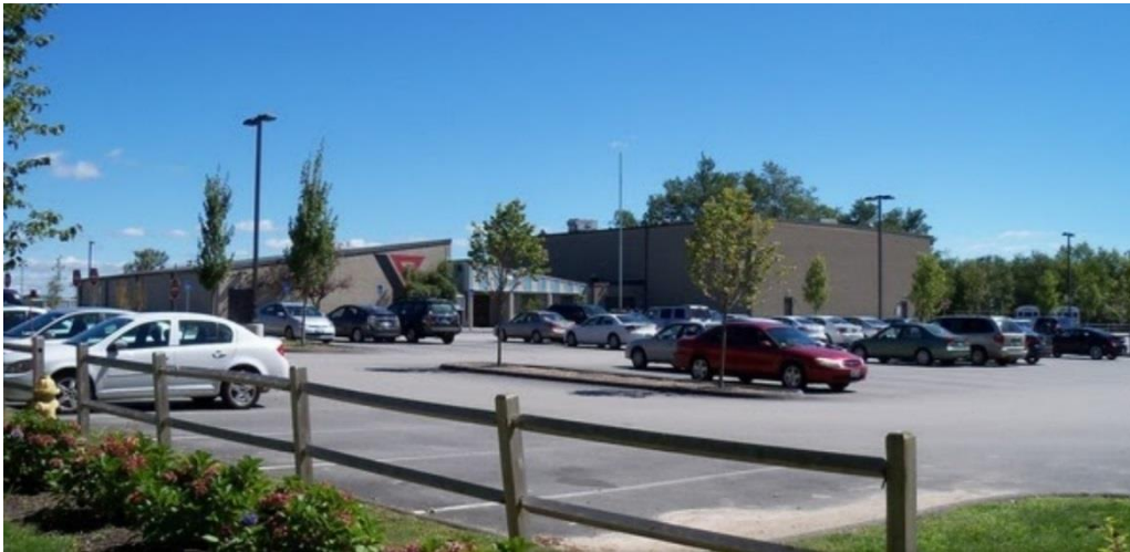
South County YMCA in Wakefield with newly converted interior/exterior LED technology lights.
