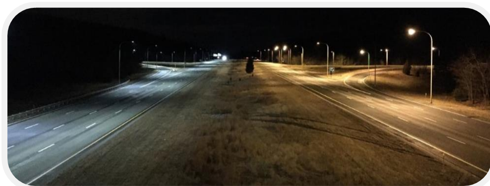
I-295 Exit 7 – Smithfield (Left side of the highway are LEDs during conversion process)
